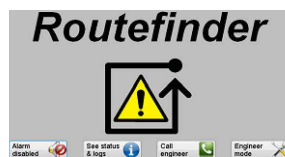
System indicating faulty status
