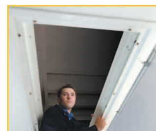
Easy Access to Ceiling Void
