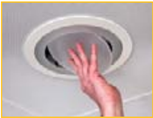
Inner Disc Installation
