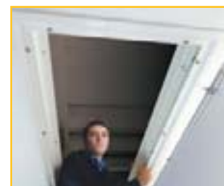
Easy Access to Ceiling Void
