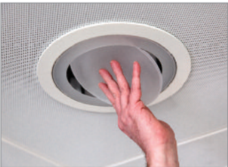
Inner disc installation
