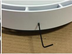
When in place use the Allen key to fix the grub screw into place and please ensure that it is flush with the surface. (Not required on IP65 variants)
