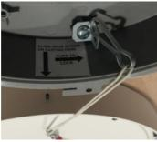
Attach the dog hook cable first to the metal bracket and then the yellow connector block(s) can now be fitted together. Connect the battery once a stable mains supply is available.
